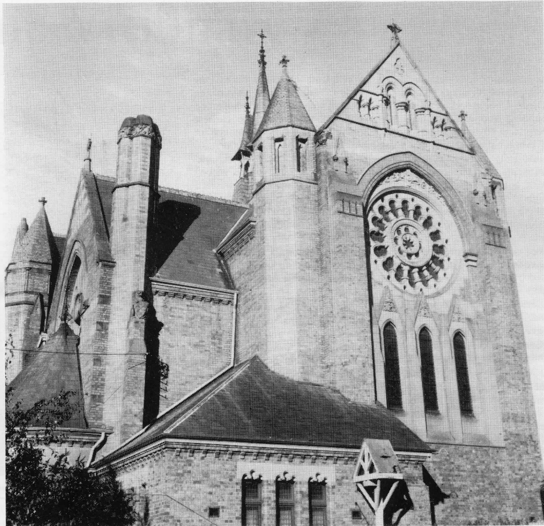
Holy Trinity Anglican Church, Launceston. East front, showing rose window, ornate decoration in gable, and fleche.
